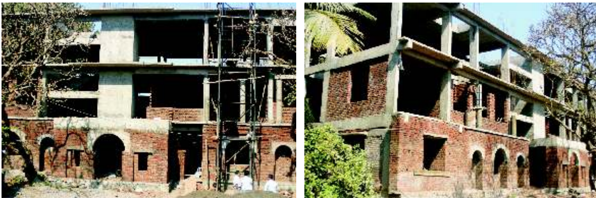
Fig. 151: Under construction students' hostel at the Bombay Veterinary College, Parel, Mumbai.
