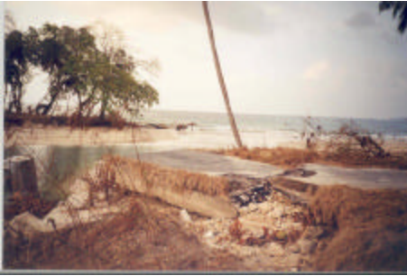
Damage due to tsunami at Car Nicobar
